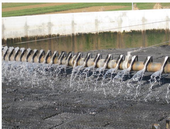
Figure 1. Trickling filter of Pogradeci WWTP (photo credit by author)
